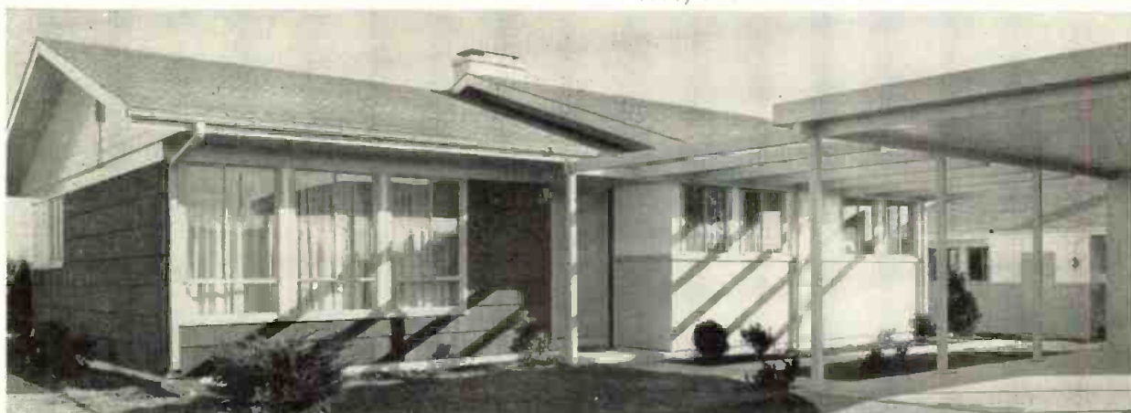
Steelaire Home. The entire structural frame of this house is made from tough, cold-formed steel, so it is unaffected by rot, fungus, and termites. Even more important is the fact that the steel frame resists warping and sagging. It's one of a line of Steelaire homes and is made by the U. S. Steel Homes Division of United States Steel.
